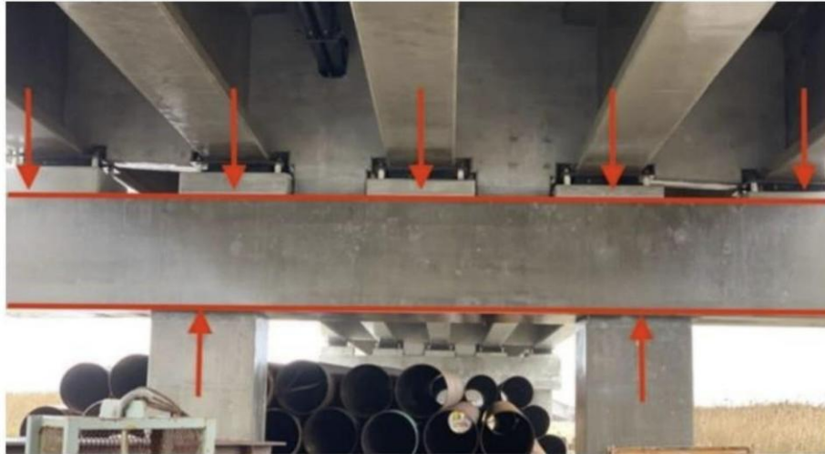
Figure A-4: Bent cap of Marc Basnight Bridge, NC, and idealization of loads.
